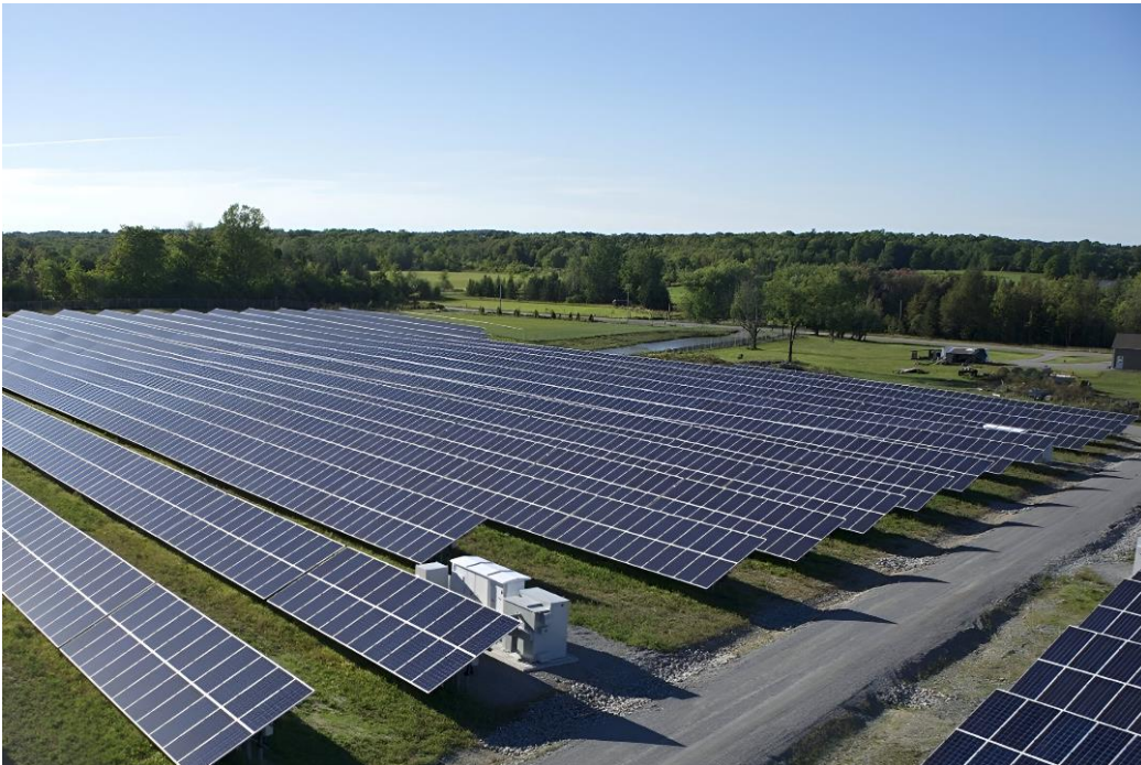
Plate 5-3 Typical fixed Solar PV Panels (with disaggregated conversion unit)
