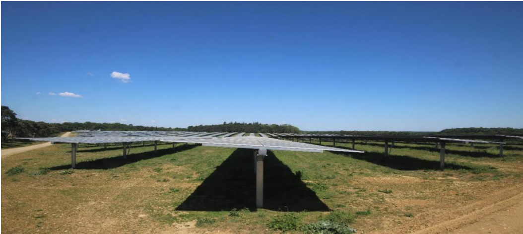
Plate 5-3 Typical fixed Solar PV Panels (with disaggregated conversion unit)
